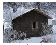
aggered fashion as one would lay bricks, locking the rows together. The window and door frames were constructed and placed as the walls went up. Sod was stuffed insulation The
