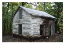
was in overall good condition, mainly because it was constructed of tamarack logs. However, the bottom three rows of logs were in poor
